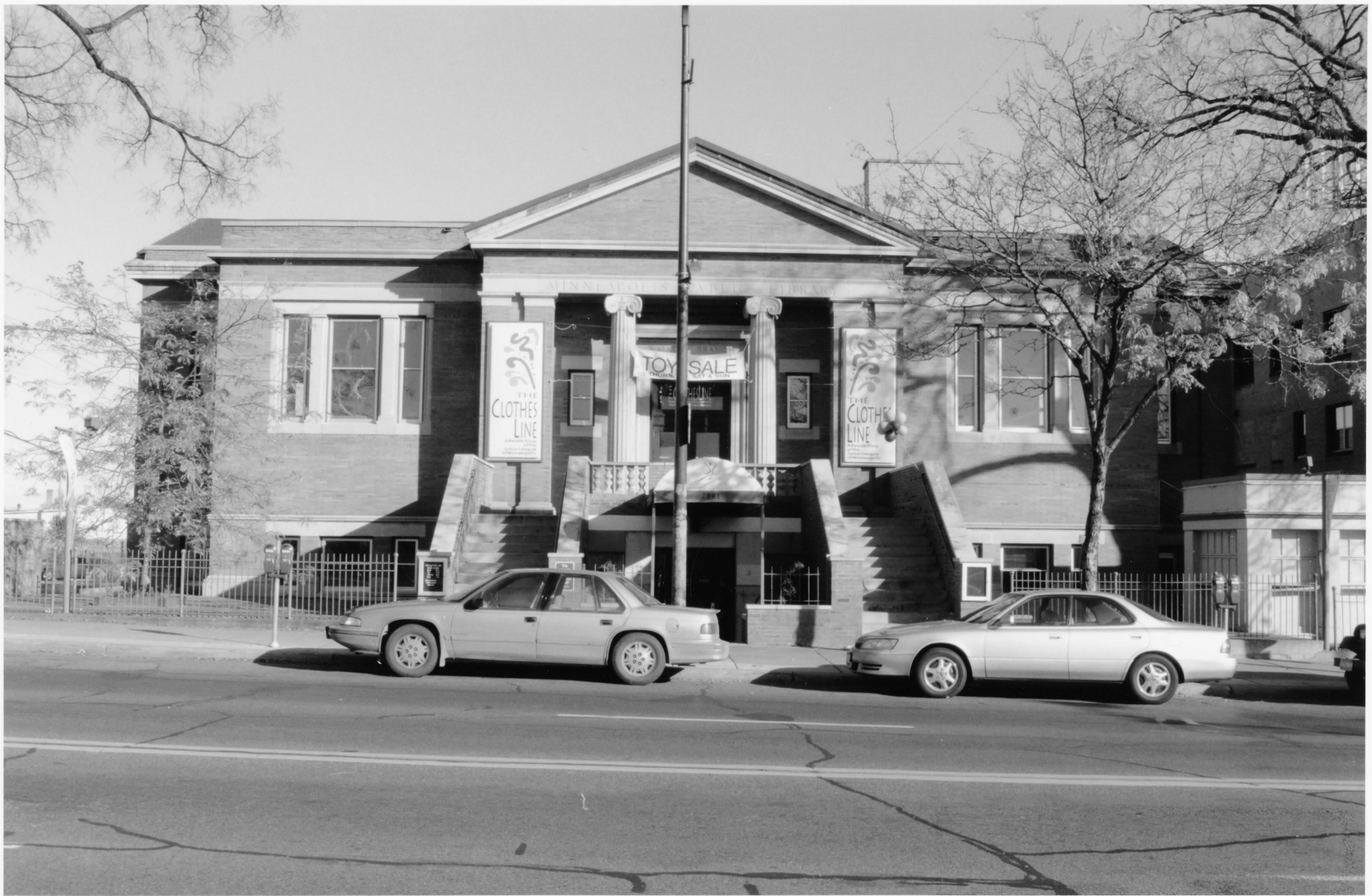
Walker Branch Library 2901 Hennepin Ave. S, Minneapolis Hennepin County, MN 013456-13
