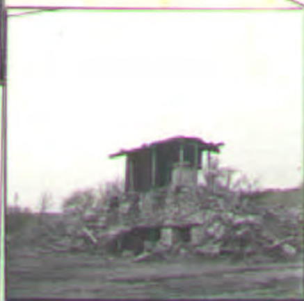
Lime Kiln, the basic foundation of which dates to General Knox's period of operation
