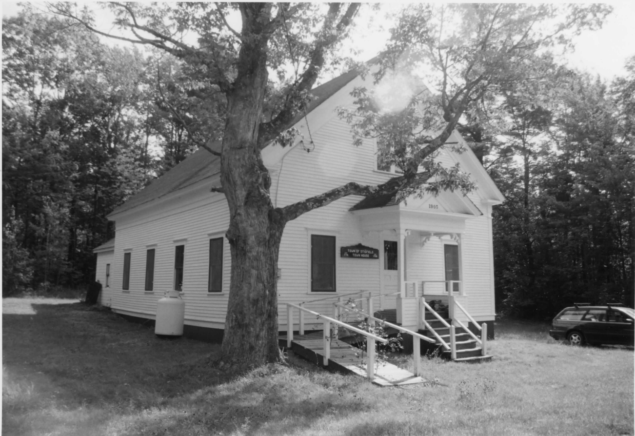
OTISFIELD TOWN HOUSE (FORMER); OXFORD CO., ME
