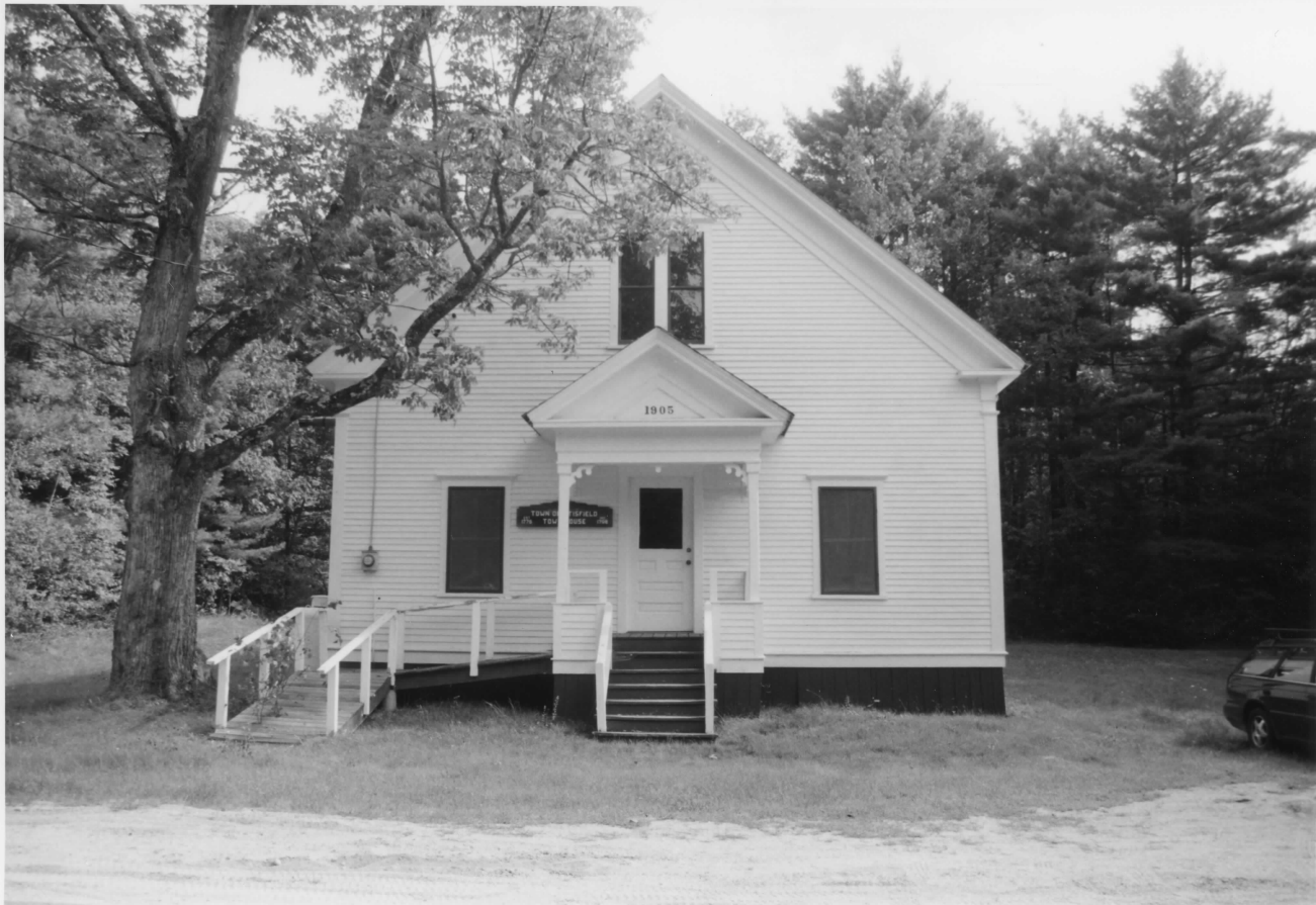
OTISFIELD TOWN HOUSE (FORMER); OXFORD CO., ME
