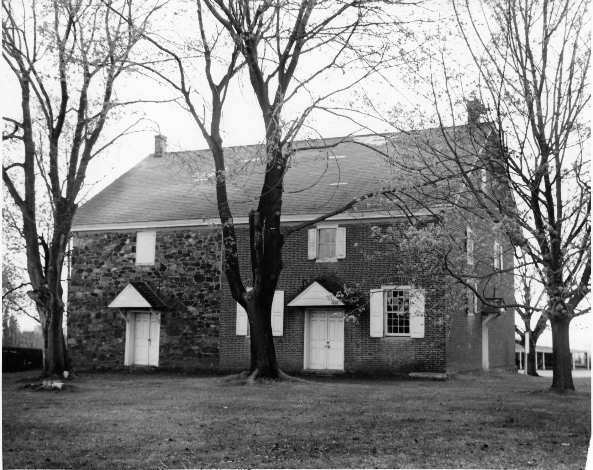
1962 before renovation FROM EAST
