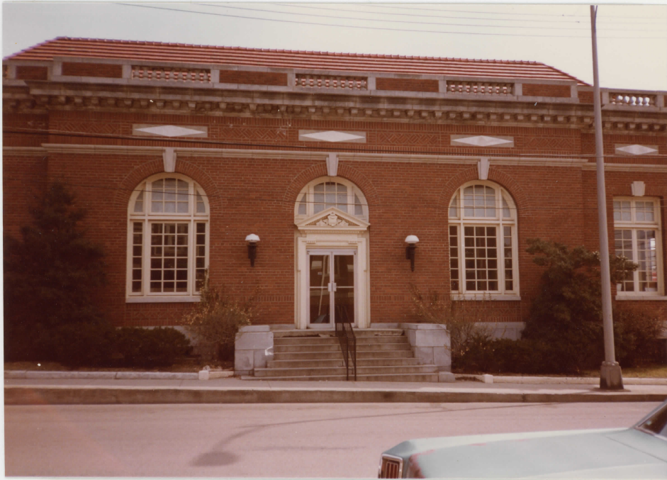
Front view of Mayfield, KY Post Office
