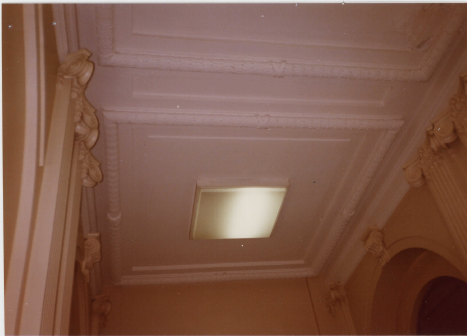
View of ceiling
