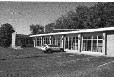
Figure 23 Potter Building 10 th Street view
