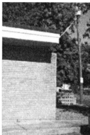
Figure 24 Potter Building Wall detail
