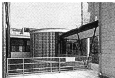
Figure 16 Drum room on another International Style Bldg.
