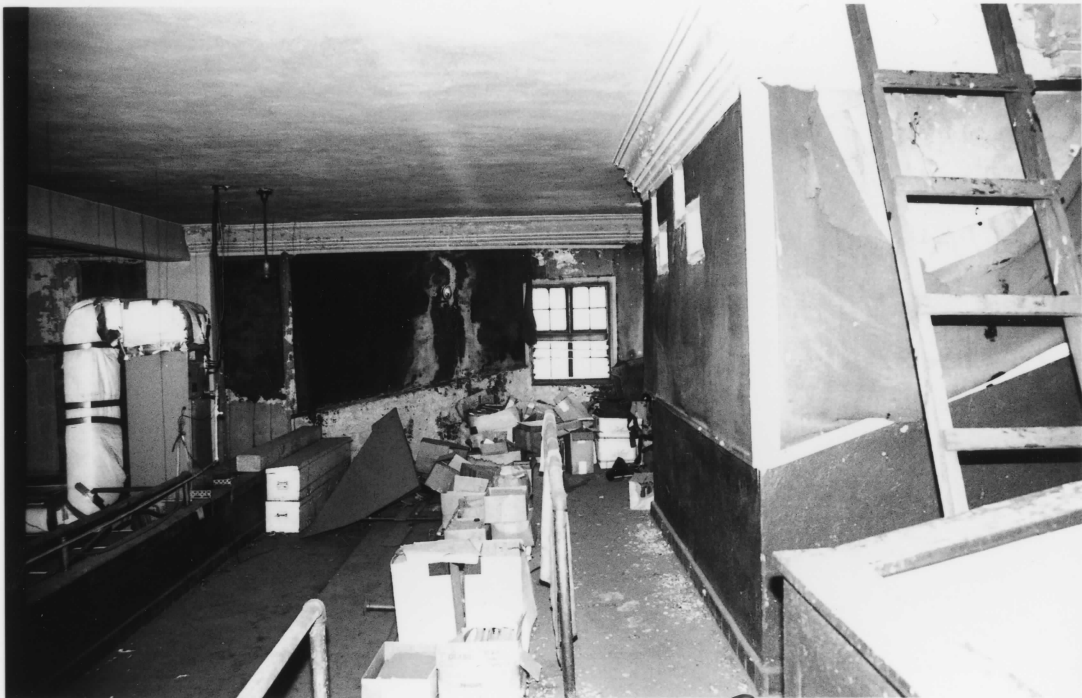
FORDSON COAL Co. BLDGS, PIKE Co, PA
