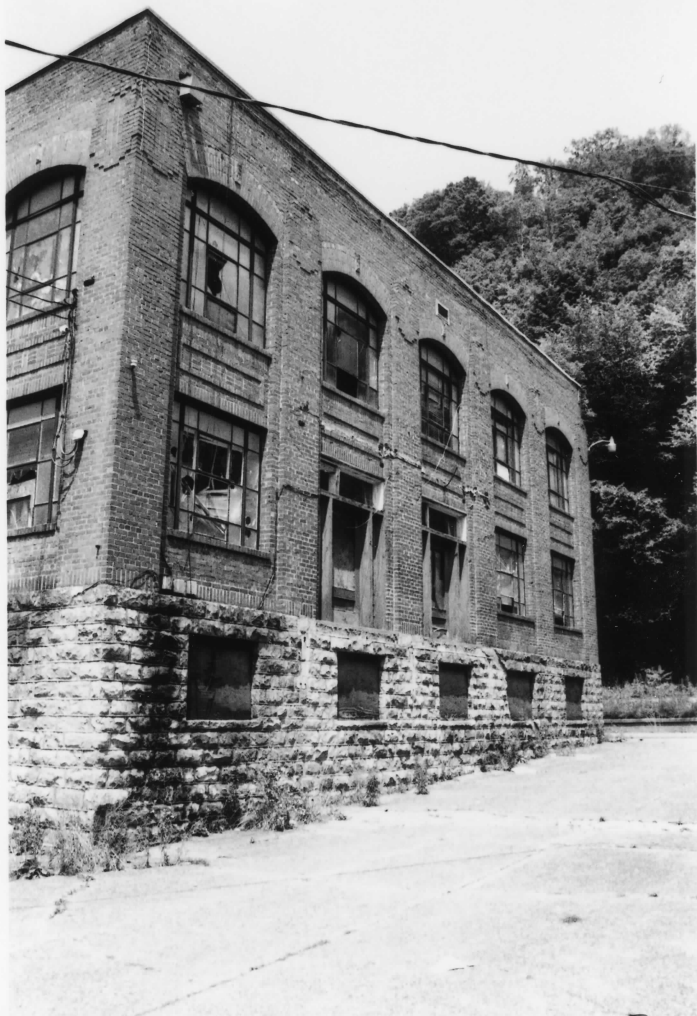
FORDSON COAL CO BLDGS PIKE CO, PA (11)
