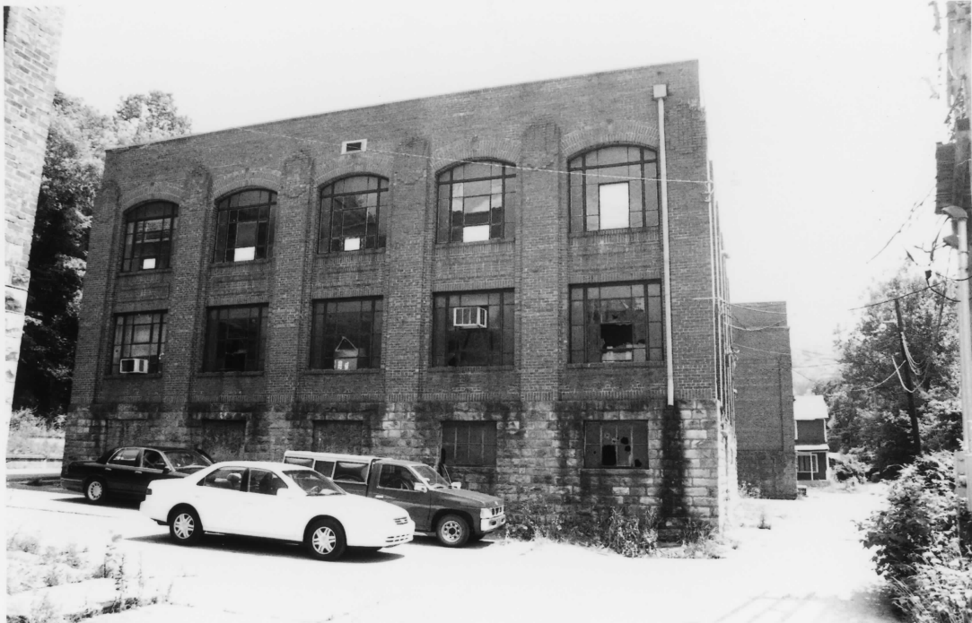
FORDSON COAL Co BLDG, PIKE Co, PA
