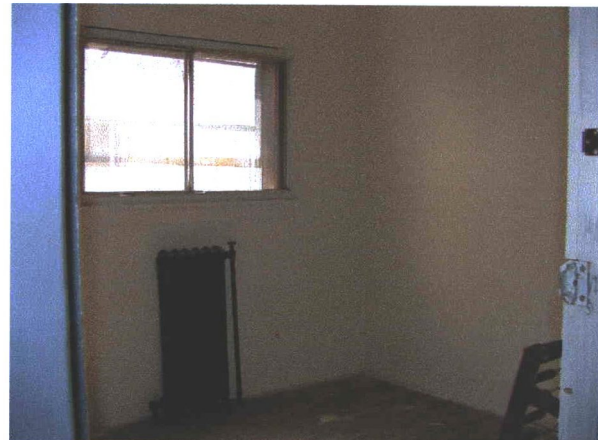
Hotel Rooms on Second Floor
