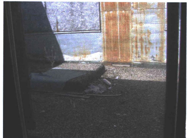
Skylight Courtyard (from Second Floor)
