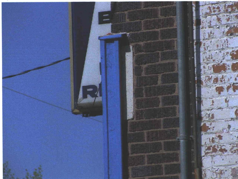
Concrete Storefront Ornamentation is in tact behind false storefront.
