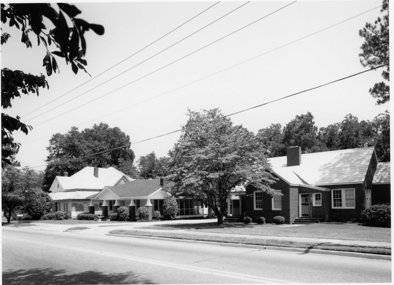
Savannah Avenue Historic District Statesboro, Bulloch County, Georgia 2 of 17
