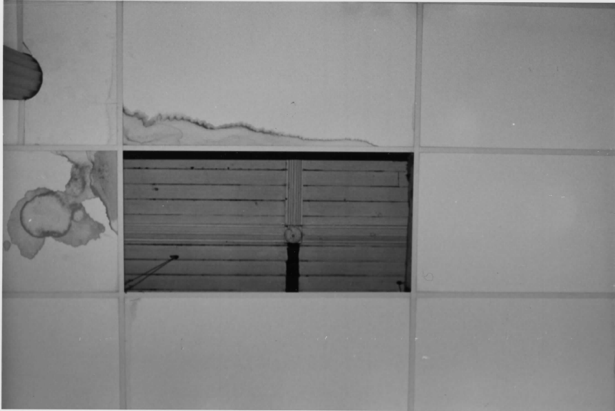
VIEW OF ORIGINAL CEILING
