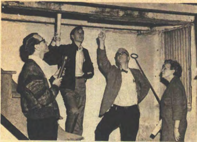
Dr. Harold Cooledge points out a massive timber which some untalented workman hacked at with a hatchet to bring these stairs down to the "new" kitchen.
