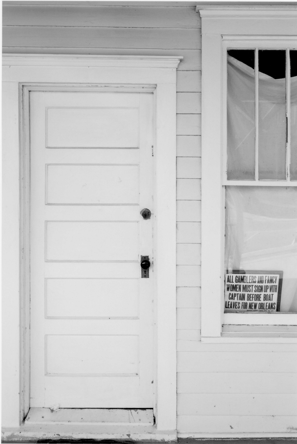
Carbo Boarding House Chatham County, Georgia Photograph 11 of 24
