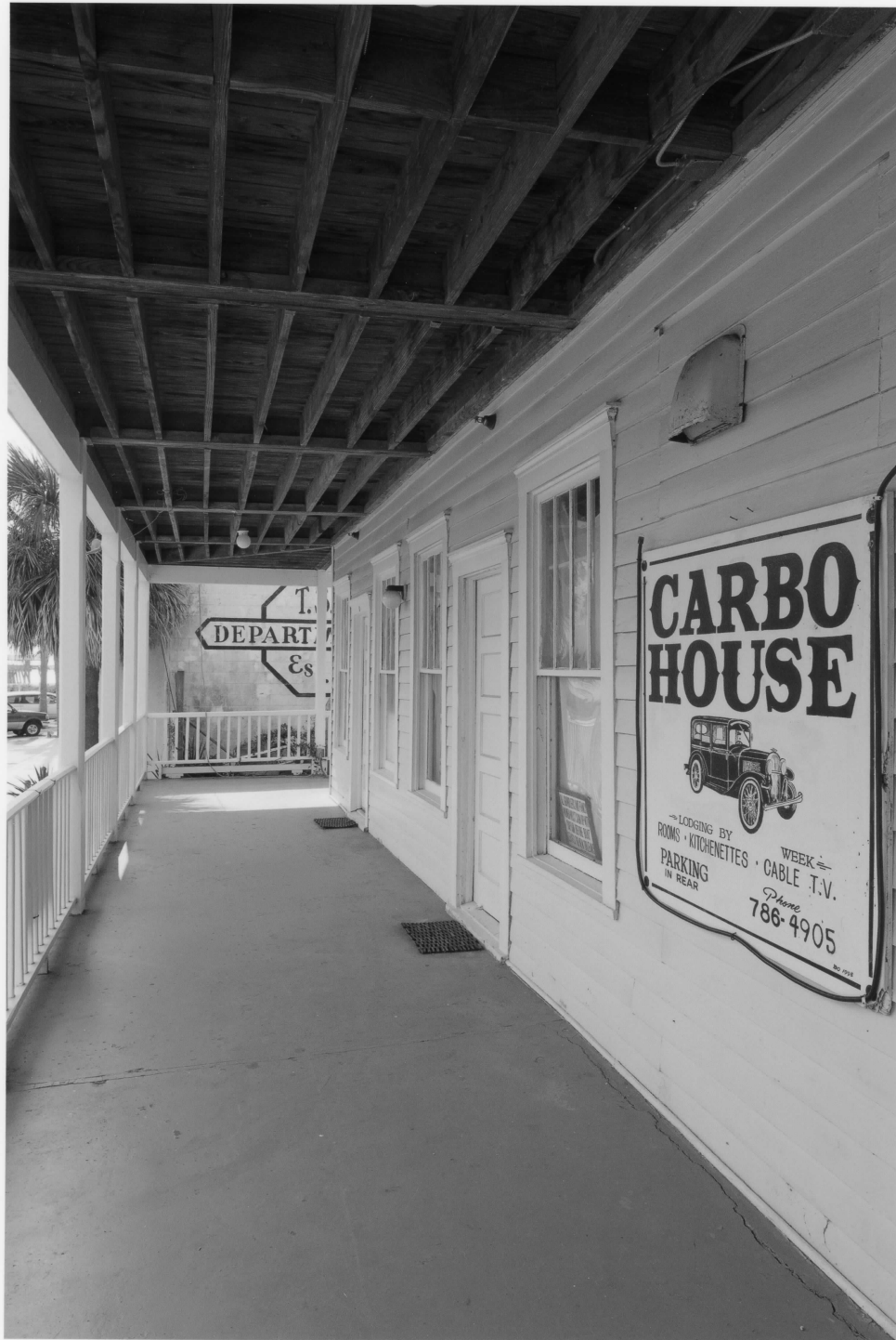
Carbo Boarding House Chatham County, Georgia Photograph 10 of 24
