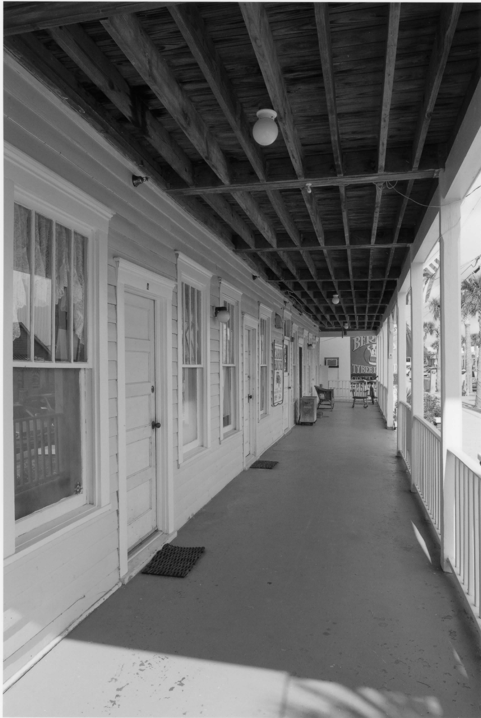
Carbo Boarding House Chatham County, Georgia Photograph 13 of 24
