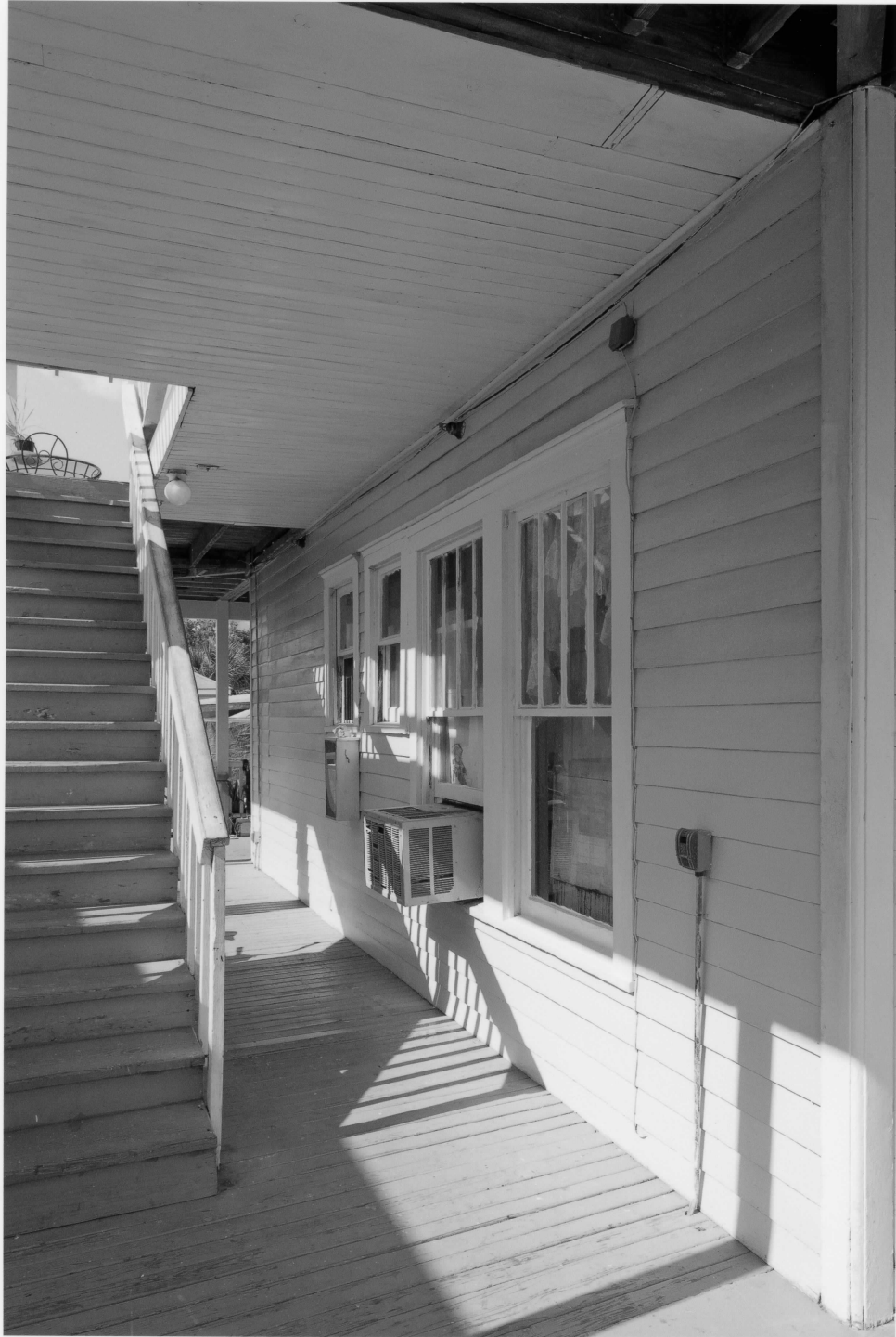
Carbo Boarding House Chatham County, Georgia Photograph 14 of 24
