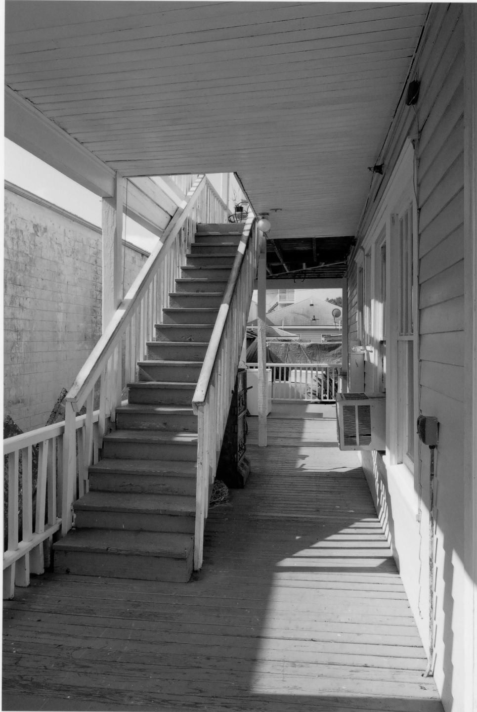
Carbo Boarding House Chatham County, Georgia Photograph 12 of 24
