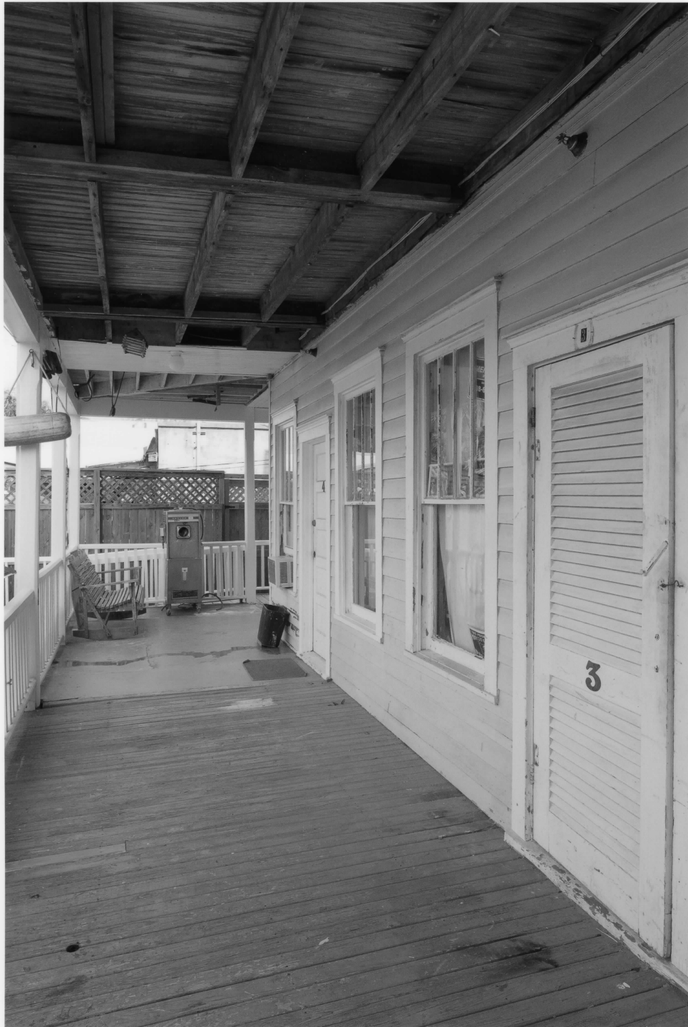
Carbo Boarding House Chatham County, Georgia Photograph 7 of 24
