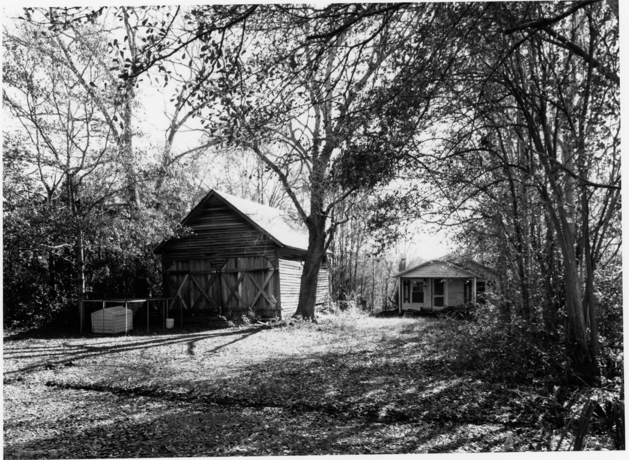
ROBERT AND MISSOURI GARBUTT HOUSE TOWNS COUNTY, GEORGIA PHOTOGRAPH 14 OF 15
