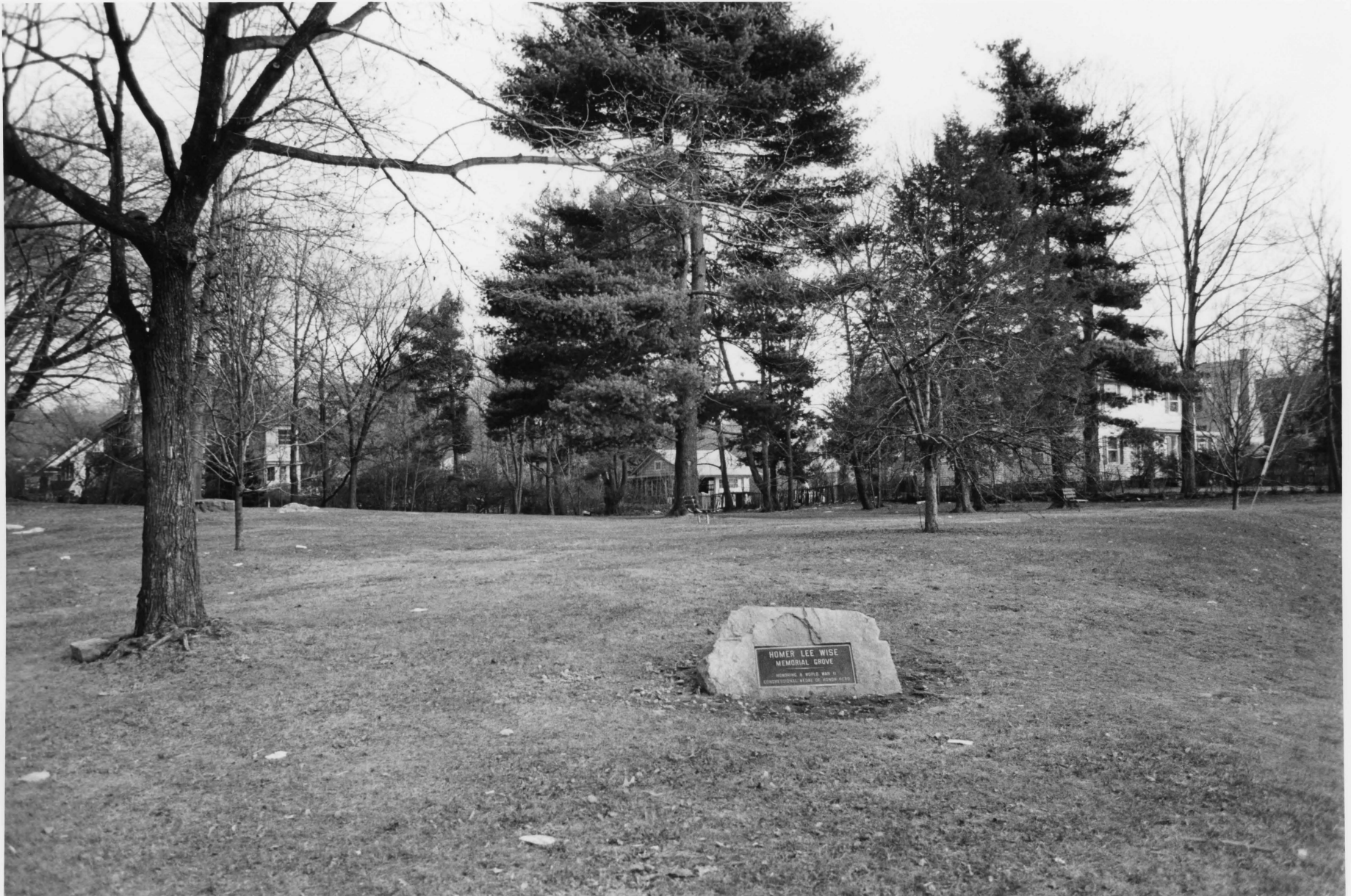
Photograph 17 Revonah Manor Historic District, Stamford, CT S. side of Chester St., E view Photo by E. Meagher. 1/86. Negatives on file with CT Historical Commission
