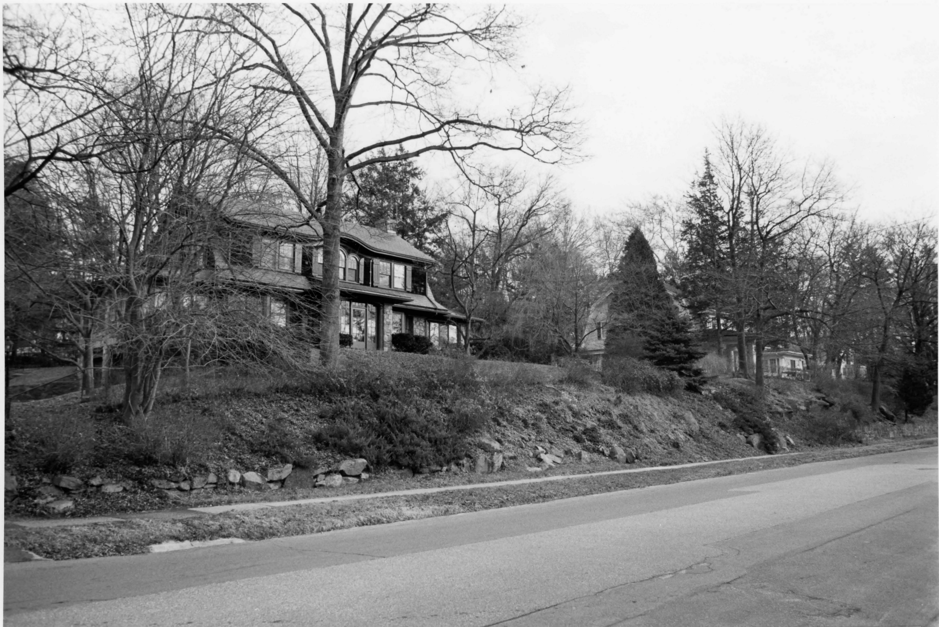
Photograph 14 Revonah Manor Historic District, Stamford, CT E. side of Revonah Ave., SE view Photo by E. Meagher, 1/86, Negatives on file with CT Historical Commission
