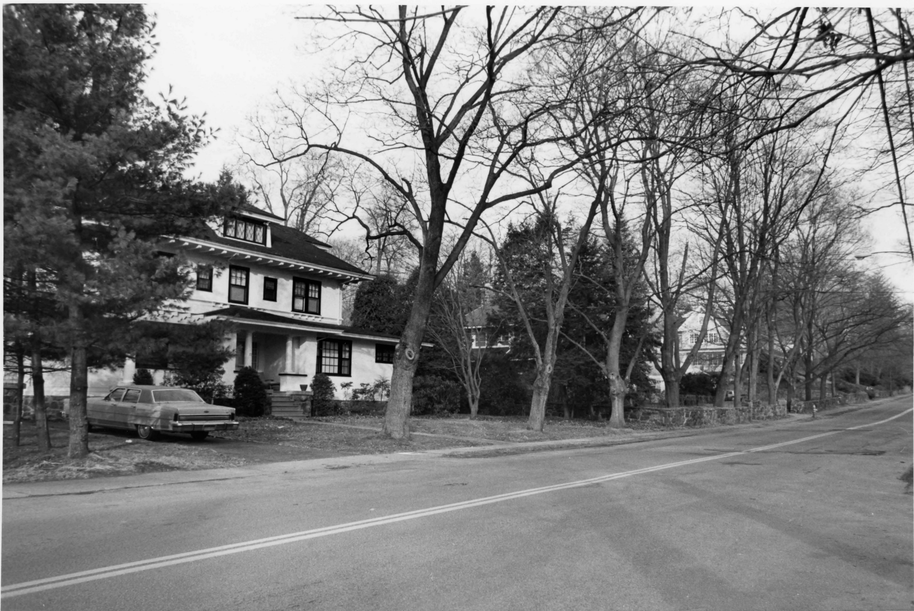
Photograph 10 Revonah Manor Historic District, Stamford, CT N. side of Urban St., NE view Photo by E. Meagher, 1/86, Negatives on file with CT Historical Commission
