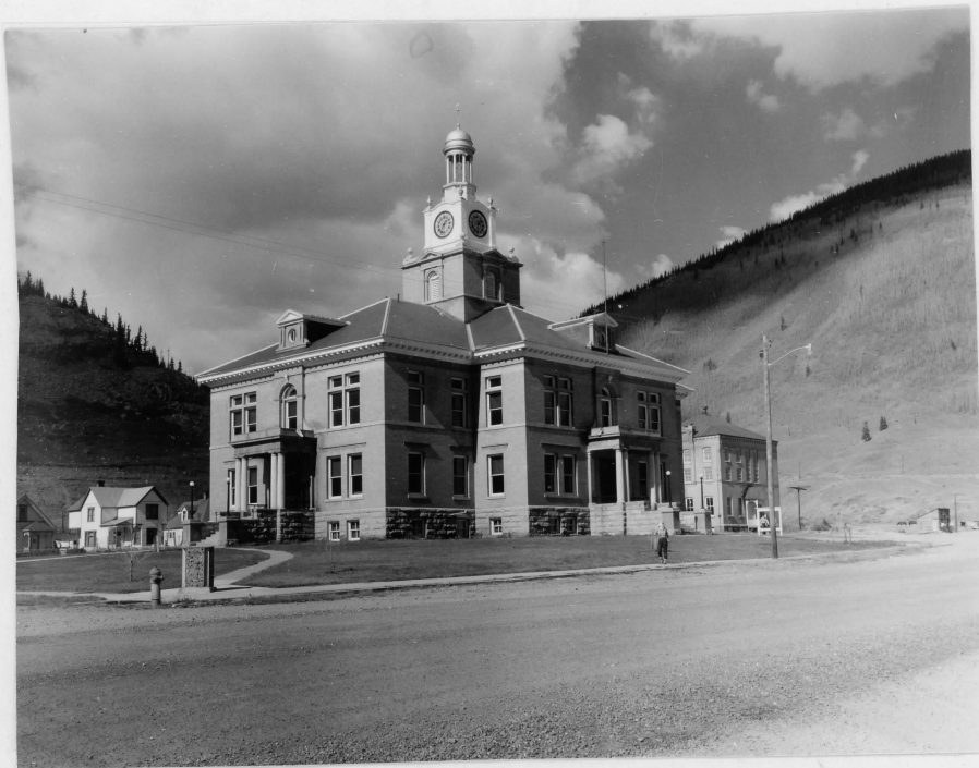
Courthouse at Silverton, Colorado, completed in 1908. Southeast view. Photograph by Ray H. Mattison, October 1958. Negative in Region Two Office Library, Omaha, Nebraska.
