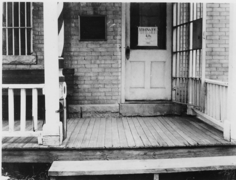
PLAQUE MOUNTED ON LEFT SIDE OF MUSEUM ENTRANCE
