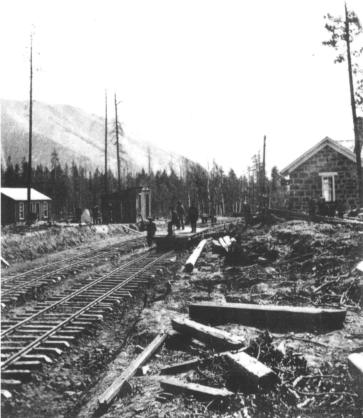
H004. Building the D&RG Railroad & Depot, 1877
