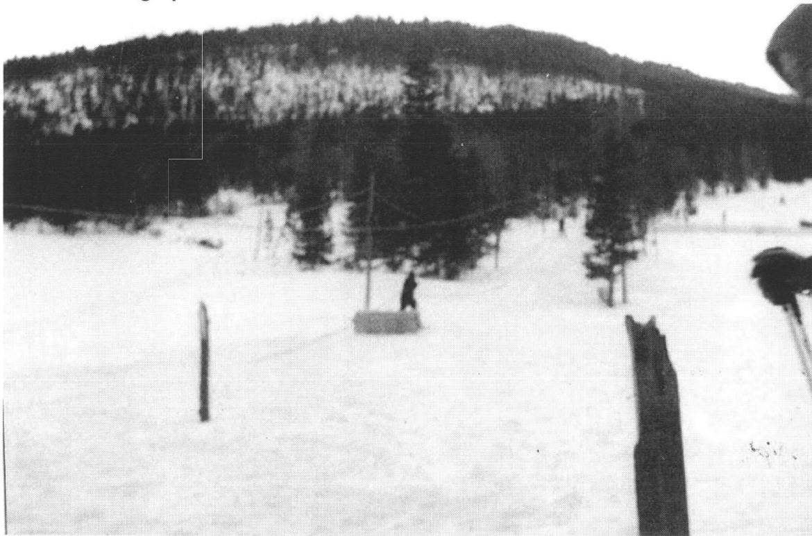
H001. Ski Lift at Uptop
