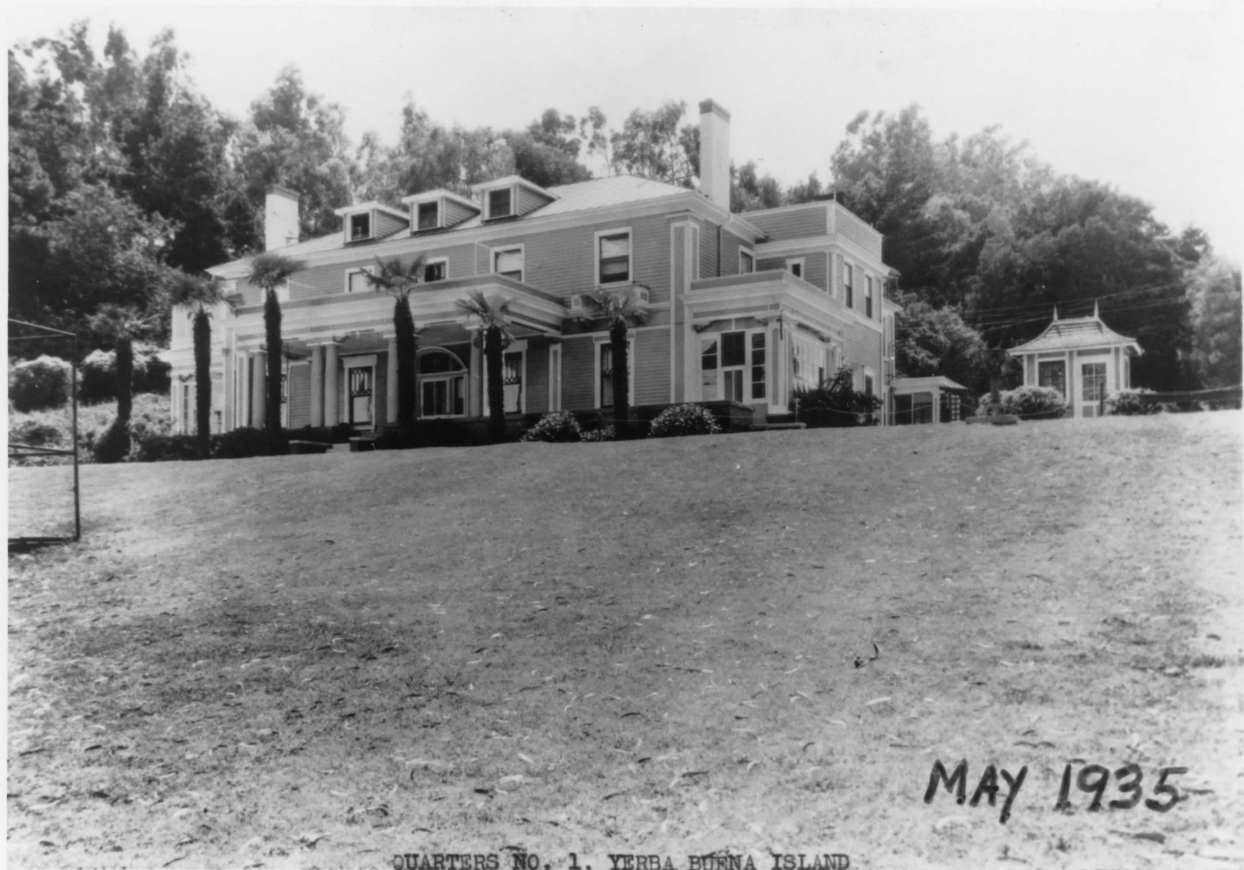
QUARTERS NO. 1. YERBA BUENA ISLAND
