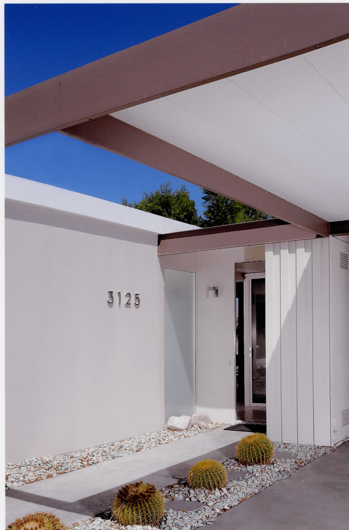
Photo 2 of 9 (CA_RiversideCounty_SteelDevtHouse2_0002) View of breezeway and entryway from carport.
