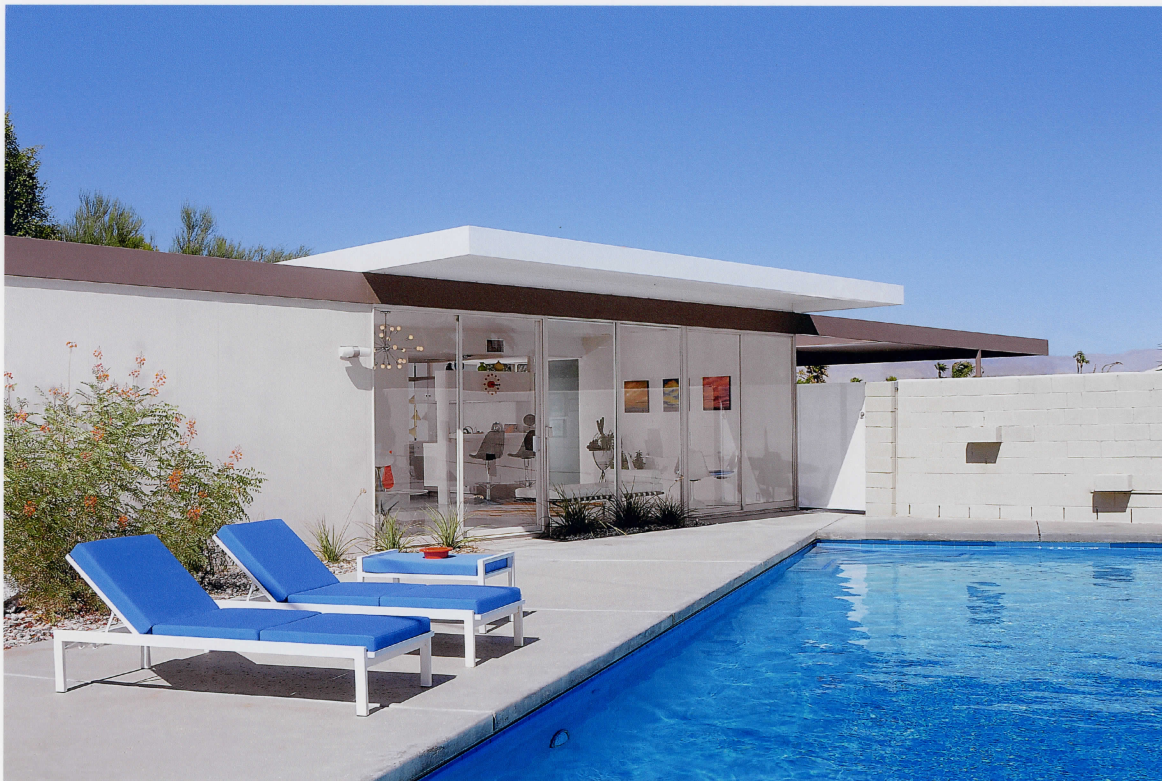
Photo 4 of 9 (CA_RiversideCounty_SteelDevtHouse2_0004) Southern elevation of the house. Note deep roof overhangs for sun protection.
