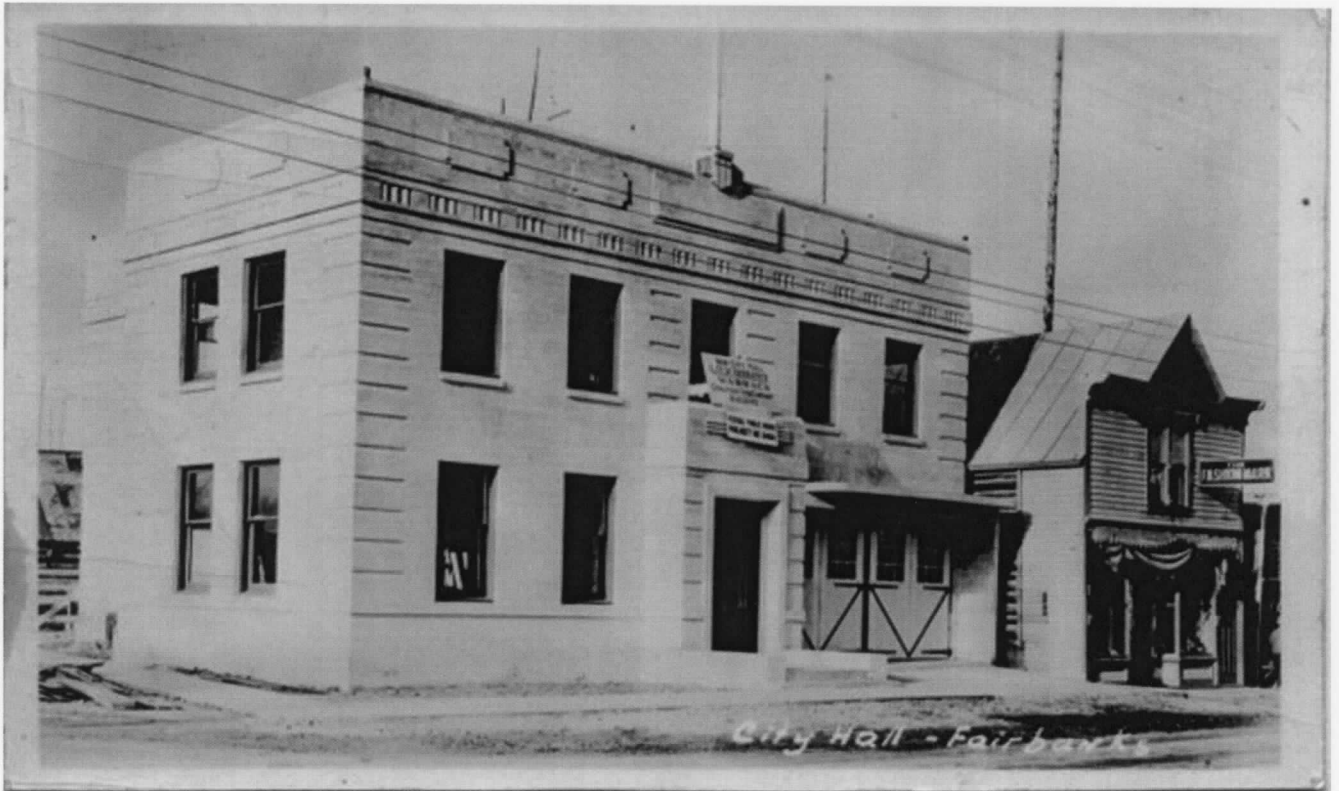
Old City Hall Fairbanks North Star, Alaska Unknown c. 1935 Candy Waugaman, P.O. Box 80589, Fairbanks, Alaska 99708-0589 Looking northwest at City Hall Photo No. 4
