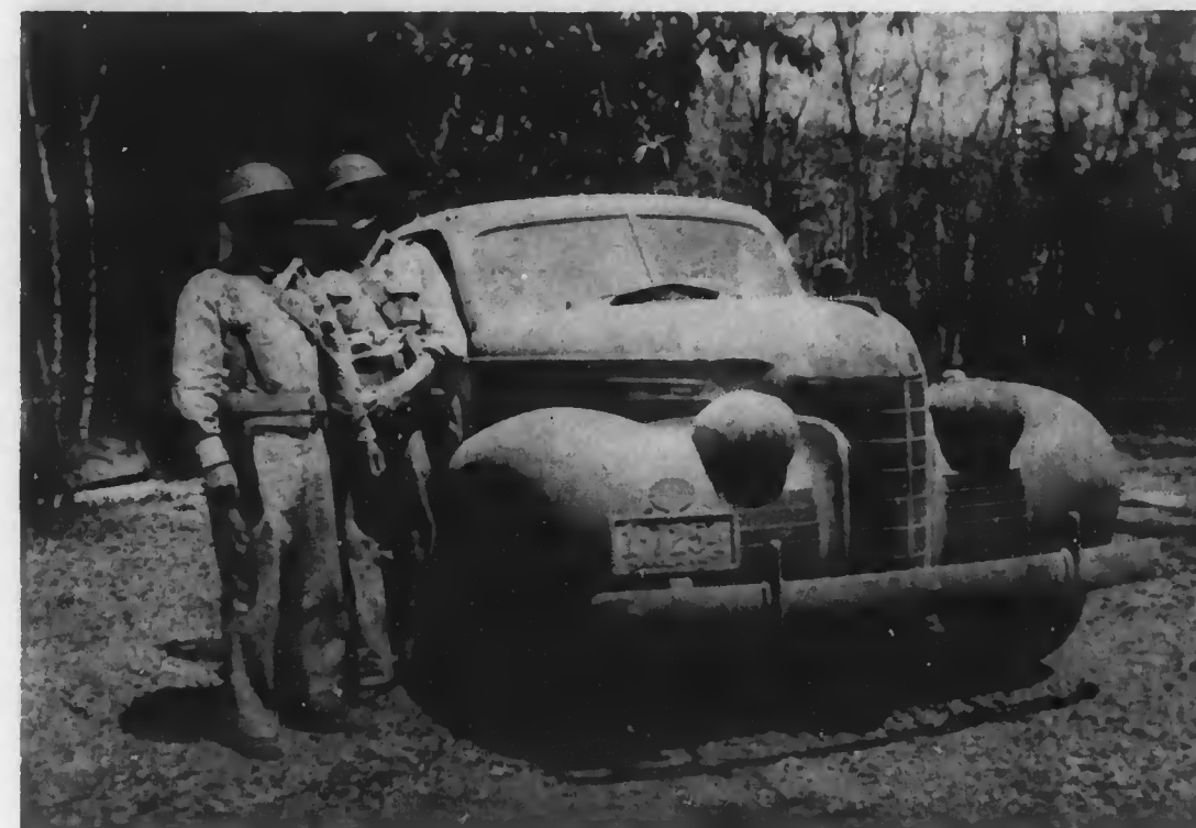
Colonel Stuart A. Hamilton, CWS, O-4663, Chemical Officer, USFIP, and 1st Lieut. Frank L. Schaf, Jr., CWS, O-396583, Assistant, on an inspection trip at Fort Mills, P. I., March 1942. The side of a Chemical Warfare galvanized iron storage shed recently damaged by Japanese air raid can be seen at left.
