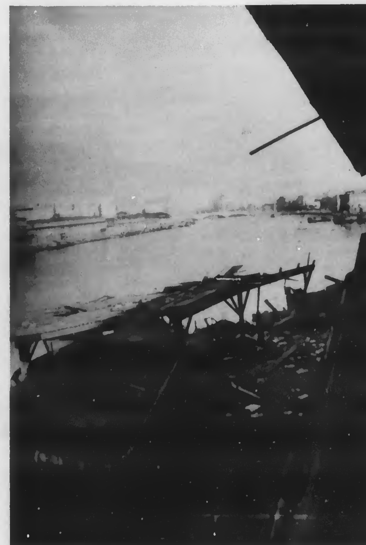
Staff officers' parking area at Headquarters Philippine Department, Fort Santiago, Manila, P. I., damaged by Japanese air raid during latter part of December 1941.
