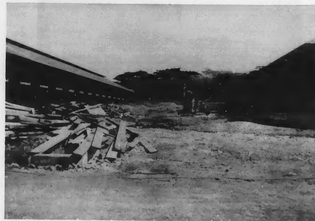
Two of the four (50' x 200') warehouses under construction at the new Chemical Warfare Sub-depot at Fort William McKinley, Rizal, P. I., when World War II started. Project was about ninety per cent complete. All warehouses with contents remaining therein were burned by Chemical Warfare details on 31 December 1941 shortly before Japanese advance elements reached the Manila Area.
