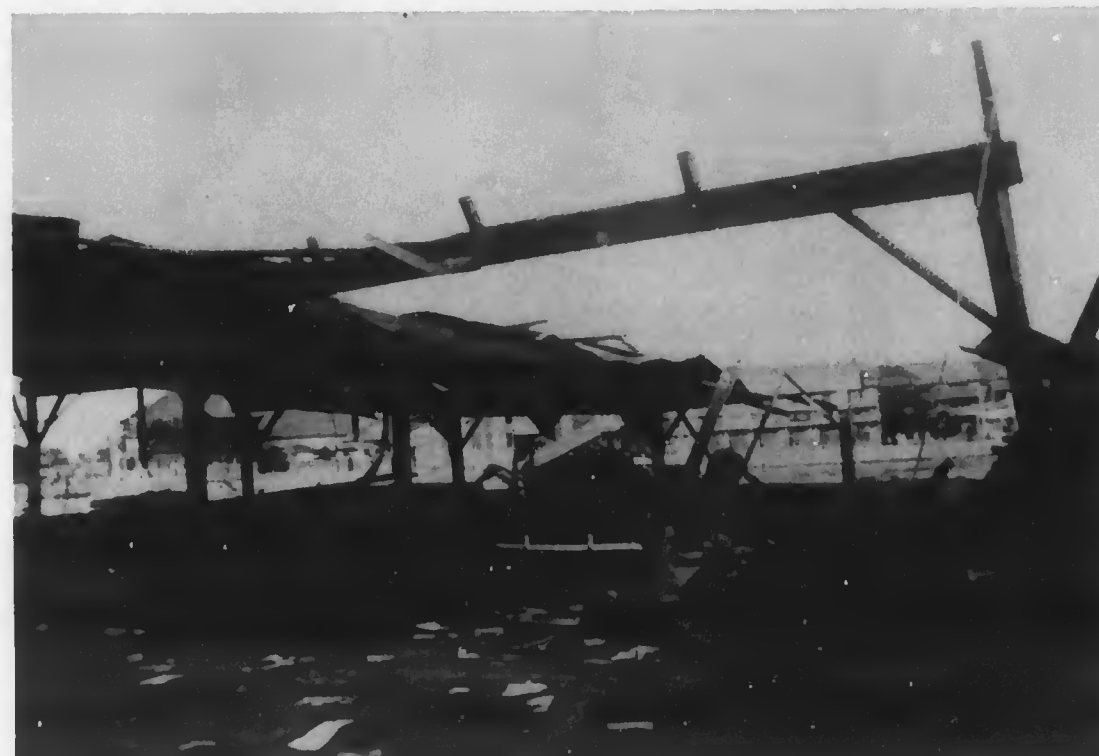
Staff officers' parking area at Headquarters Philippine Department, Fort Santiago, Manila, P. I., after a Japanese air raid during latter part of December 1941.
