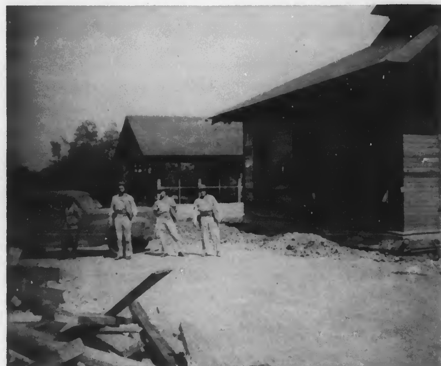
One of the four (50' x 200') warehouses and the motor vehicle shed which were under construction at the new Chemical Warfare Sub-depot at Fort William McKinley, Rizal, P. I. in December 1941. Personnel right to left:
