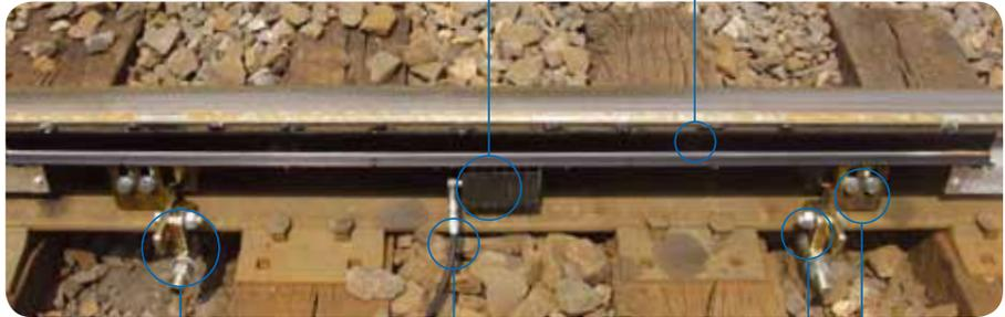
*Upgraded brackets allow for easy reinstallation after rail grinding.*
