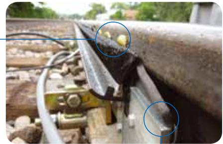
*Wiper bar is tucked under the rail to eliminate wheel strikes.*
