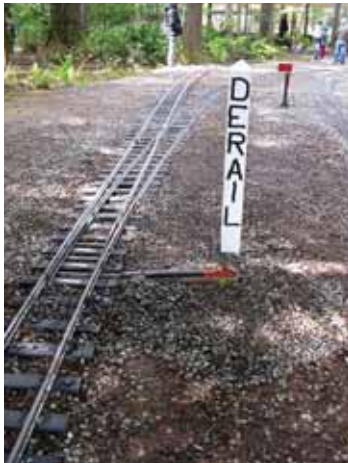
A 4 x 4 has been added to keep the members from tripping
