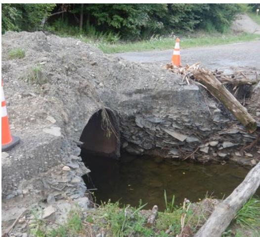
*Undersized culverts can be washed over by high waters, eroding the surrounding infrastructure and sending debris downstream.*
