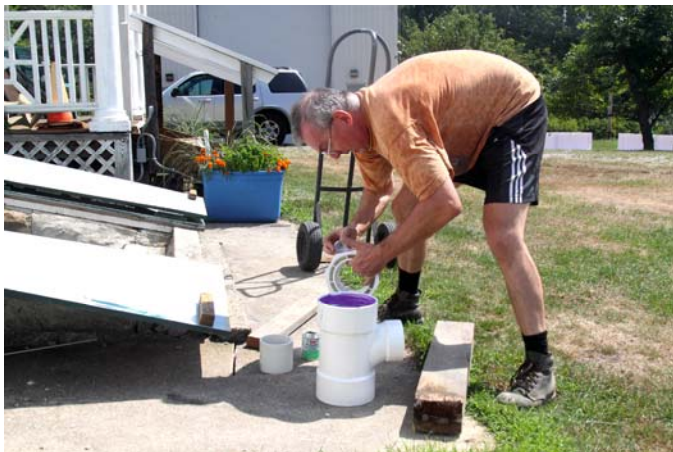
Slav Mlch preparing the new drain system piping. *
