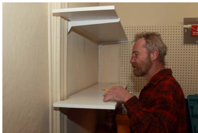
Dave Prowten installing shelves in the Telescope Room *
