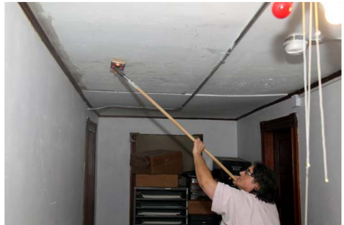
Maria Batista working on the 2nd floor hallway ceiling. *
