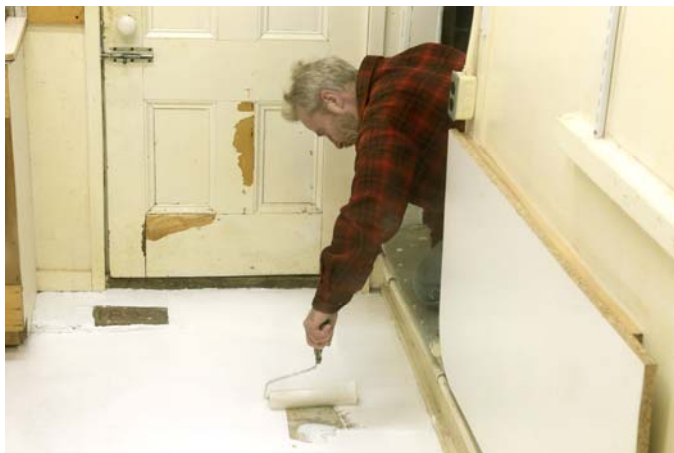
Dave Prowten painting the former Evaporator Room floor *
