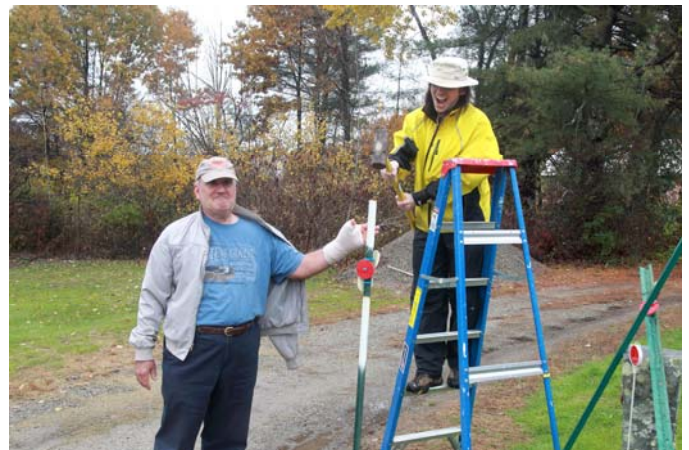
(L-R) Paul Cicchetti and Chris Elledge installing the "snow fence" *
