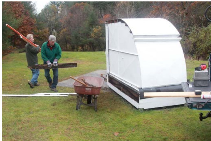
(L-R) Dave Prowten and Steve Clougherty repairing the Chase Hutch. *
