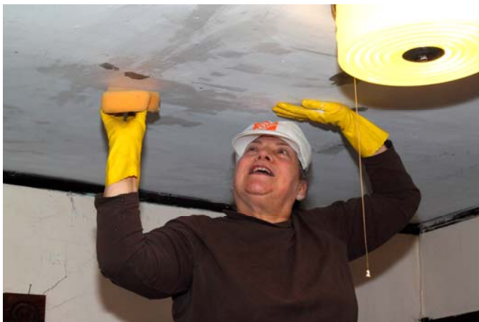
Marsha Bowman prepping the ceiling for painting *
