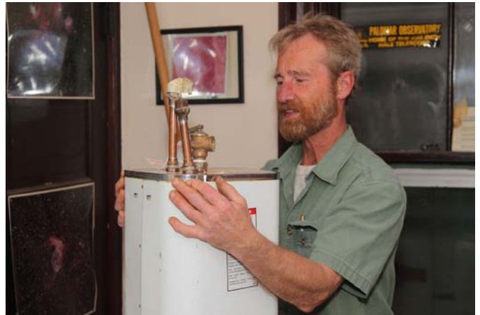
Dave Prowten installing the water heater *
