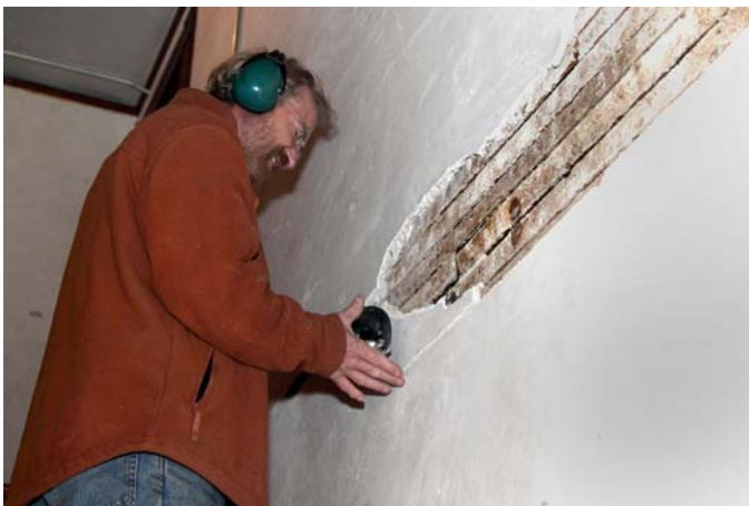
Dave Prowten working on the stairwell plaster wall.. *
