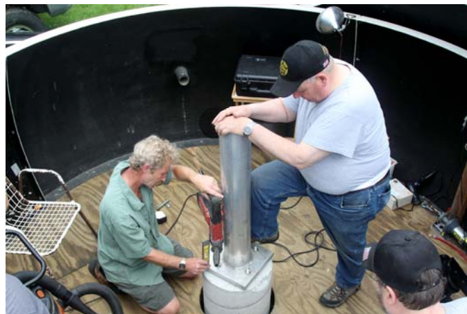
(L-R) Dave Prowten, John Blomquist and John Maher installing the G-11 pier. *
