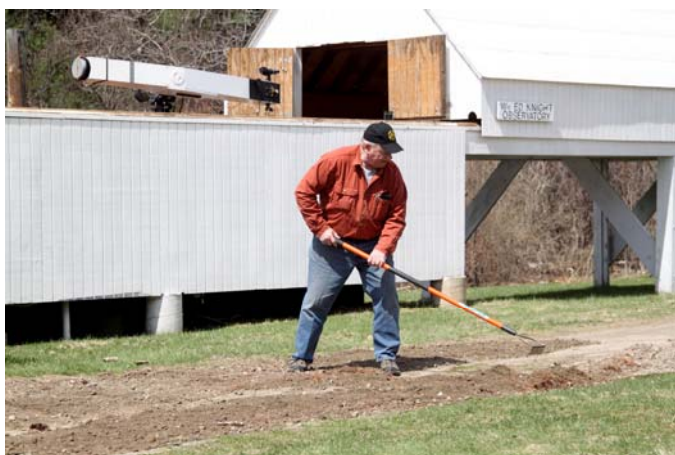
John Blomquist leveling packer material on the driveway. *
