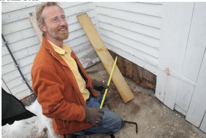
Dave Prowten fixing the barn sill. Image by Al T.
