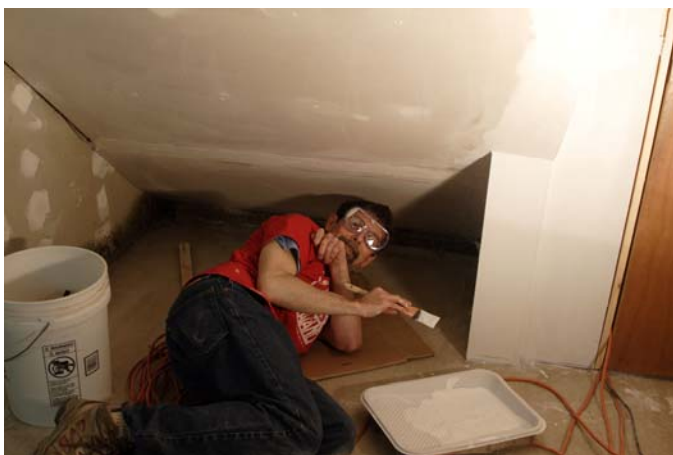
Mike Hill painting the future machine shop. Image by Al Takeda
