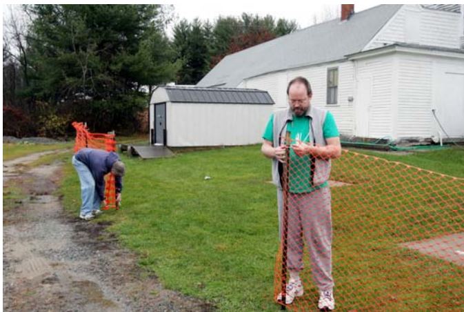
Installing the snow fence. (L-R) Dave Siegrist, and Eric Johansson. Image by Al Takeda
