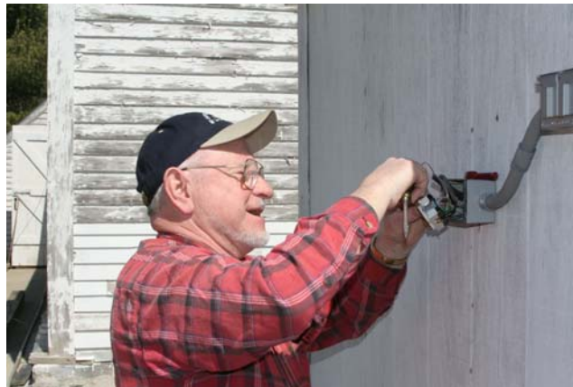
John Reed installs a new electrical fixture at the Clubhouse
