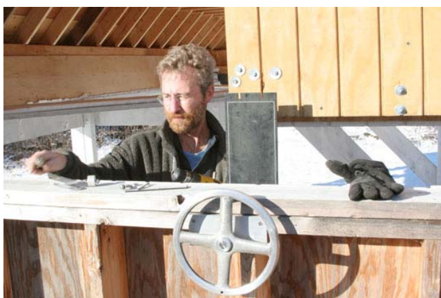
Dave Prowten installs the new roof latch. Image by Al Takeda
