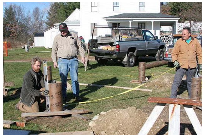
Dave, John and Paul prepare the forms for the concrete pour
