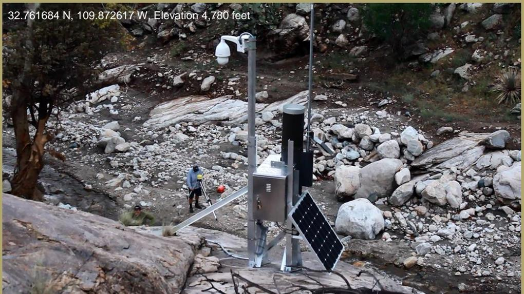
JE Fuller finished installing this new combination ALERT precipitation/stream and PTZ camera station on September 14<sup>th</sup>, 2017. This station was installed to provide advance indication of flooding from the Ash Creek Watershed which was recently burned by the Frye Fire that consumed over 48,000 acres in the Pinaleño Mountains of Arizona. Real-time data and camera imagery collected by this station can be accessed at <https://water.azgfd.gov>.
