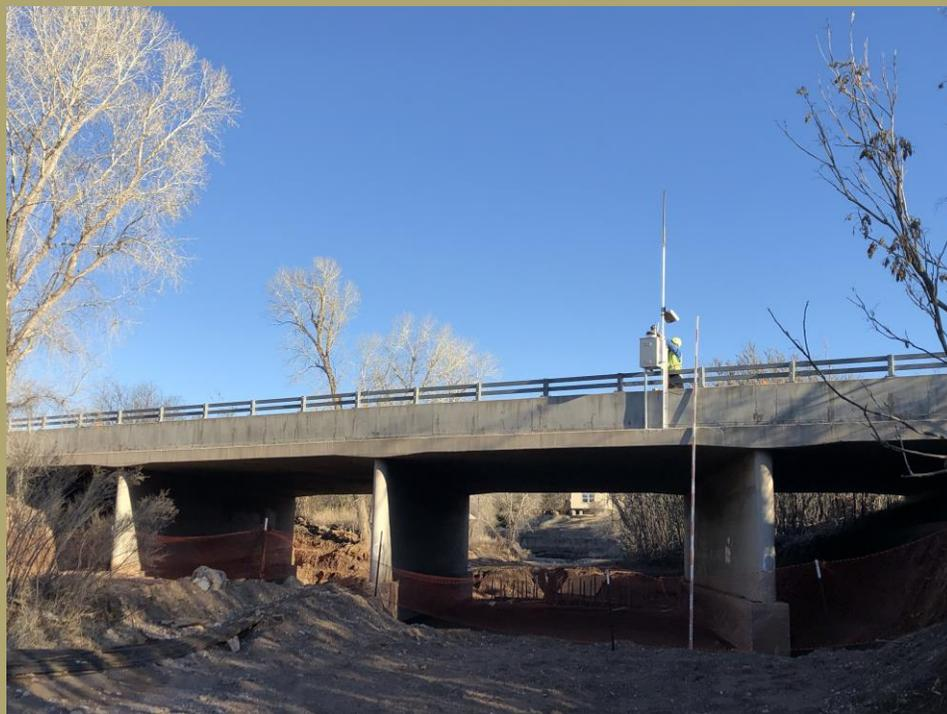
The Santa Cruz County Flood Control District, Arizona installed this new ALERT precipitation/stream station on Sonoita Creek in Patagonia Arizona on February 13<sup>th</sup>, 2020. This station features a radar sensor for measuring stream stage. Realtime data may be viewed at <https://santacruz.jefulleralert.com/>
