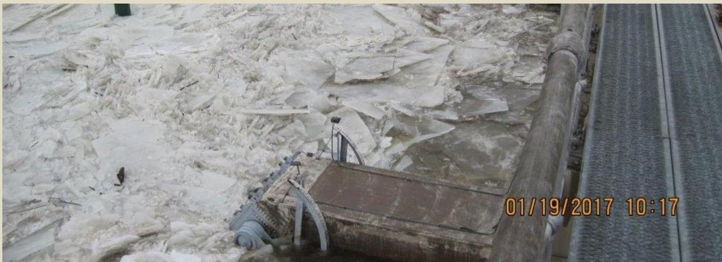
Ice locked in place at Lock & Dam 18 on Jan 19, 2017. A 6-foot shift and backwater due to ice caused major flooding in the Burlington, Iowa area. Photo credit: USACE, Rock Island District
