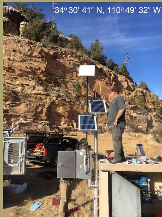
This remote dam, owned and operated by the Arizona Game and Fish Department, had inoperable principal outlet valves and no way to control the actuator remotely. Without a way to monitor lake level and control the principal outlet valves remotely, it was necessary for Department employees to travel several hours to the dam to assess hydrologic conditions and manually actuate the valves.
