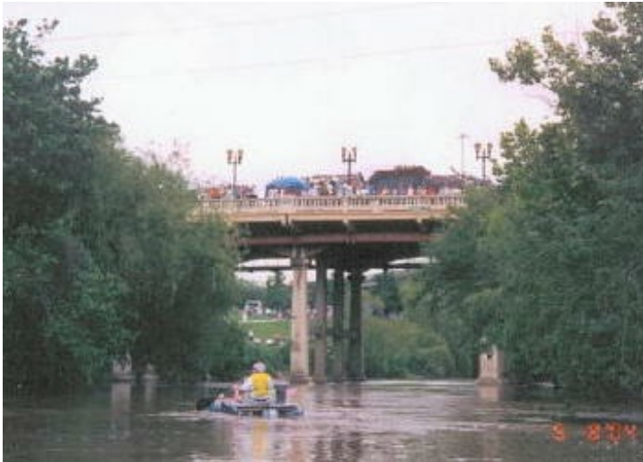
Sabine Street Bridge
