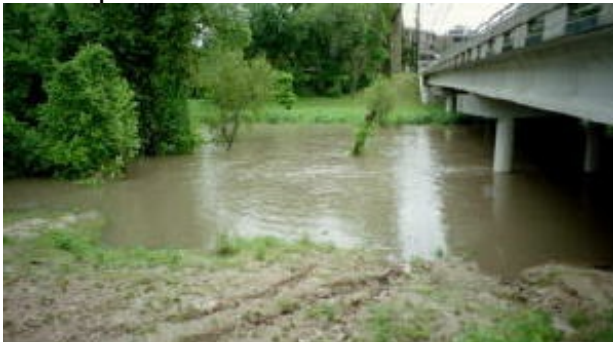
Woodway Launch Site
