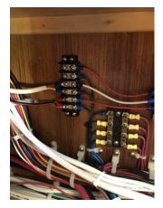
A 14 AWG 2-wire safety marine cable was installed for the Axiom +9. The cable terminates in the 6-way junction block above the SeaTalkNG power cable. 14 AWG black wire (DC -) was led to the negative bus on the distribution panel and 14 AWG white wire (DC +) was led to a 7.5A ATC fuse and then to a 10A thermal breaker on the distribution panel.
