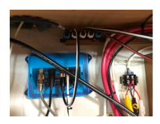
Due to the size of the spur cable (A06045) leading from the Vesper Marine XB-8000 AIS device to the 5-way back bone connector, I had to relocate the AIS device. I took the opportunity to install a 3A in-line fuse to the AIS splitter and do some cable management for the power going into and out of a 2-way junction block so that all three fuses were in the same location. The in-line fuses from left to right are: 3A – AIS splitter; 3A – AIS power and 10A – VHF power.
