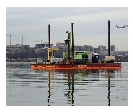
Construction activities consist of drilling geotechnical borings and collecting subsurface information in the Potomac River between the Potomac Boat Club and Thompson Boat Center Dock. Boring work will include advancing 9-inch diameter boreholes into the ground and collecting soil and rock samples and in-situ testing.
