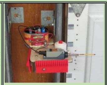
The first step was to build a platform to hold the limit switch, alarm and battery pack. A piece of ¼ inch plywood was cut to the shape required. A metal "L" bract was attached to the platform and then screwed into the wood panel between the doors.
