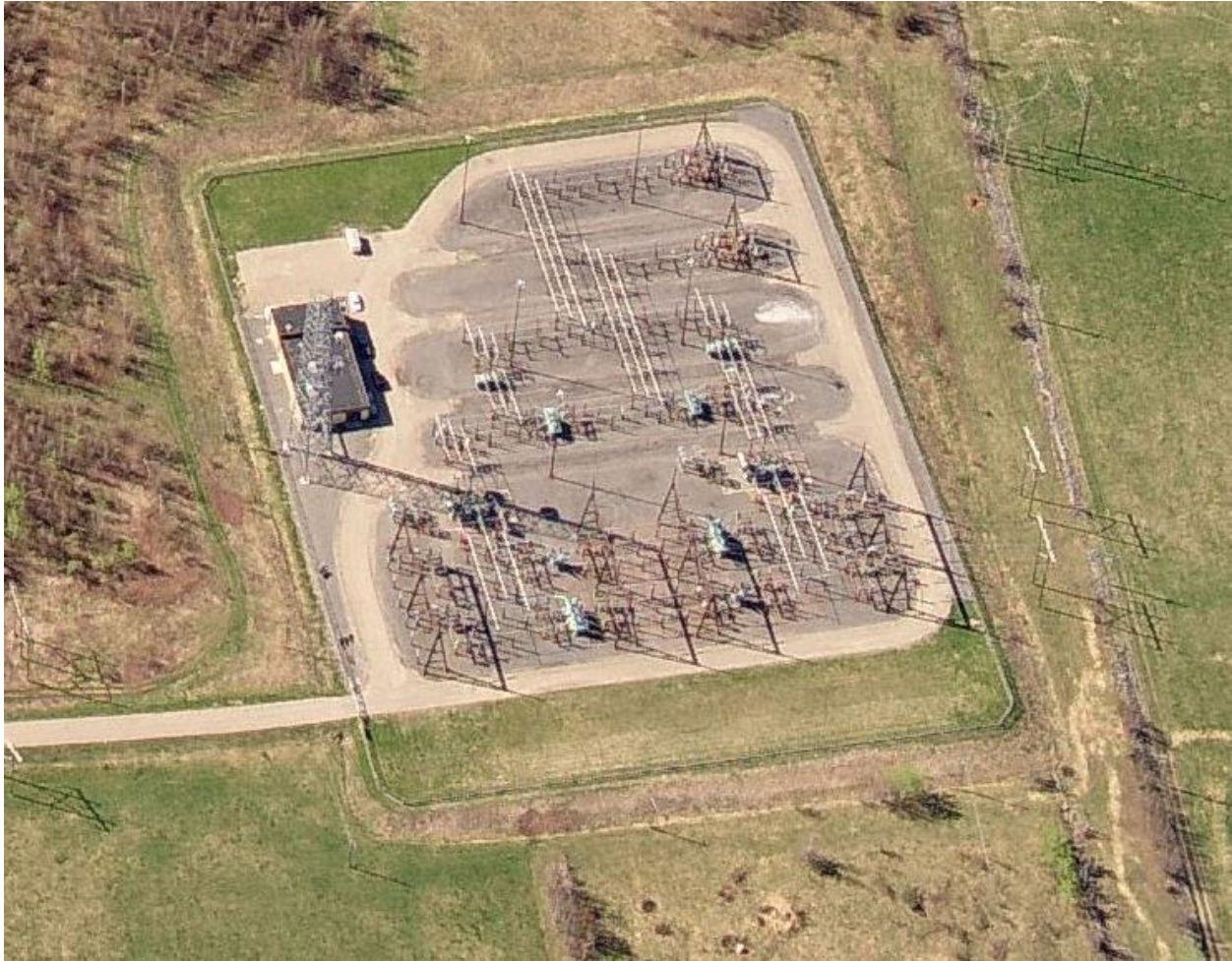
Figure 2: Aerial View of Tower in Substation Facing South
