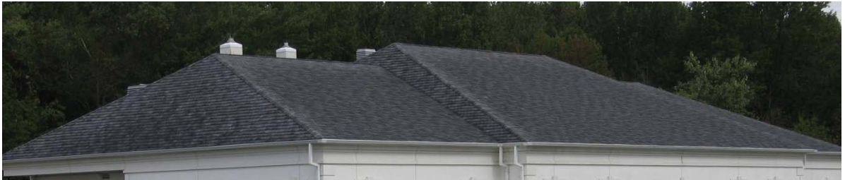
Asphalt shingle roof
