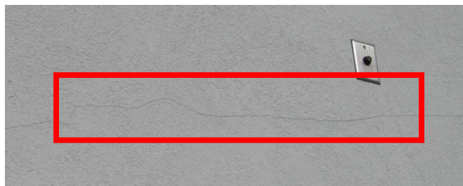
Crack in stucco facade
